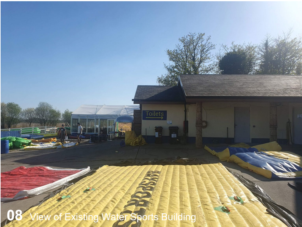
The Existing Water Sports Operator building is a single-storey blockwork structure with yellow rendered walls and a series of pitched roofs. It is located centrally within the site and is surrounded by a hard concrete terrace.
